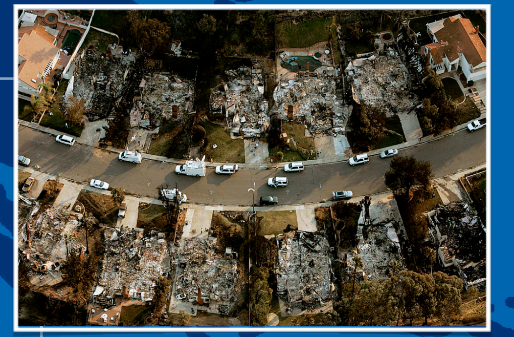
Destroyed housing in San Diego County following the Rice Fire (ImageCat, 2007)
